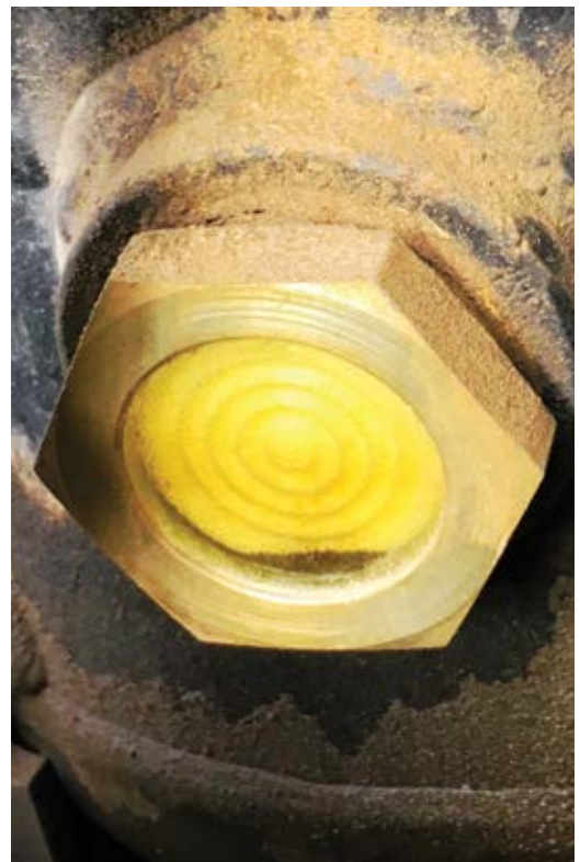
Fig. 4: A sight glass or filter plug are provided to check compressor head lubricant level
