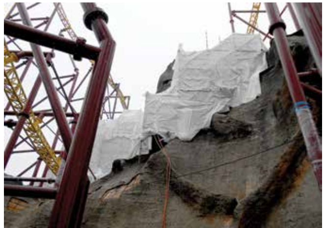
Fig. 12: Scaffolding and the plastic protection over the mountain areas to be repaired Photo by Ray Schallom
