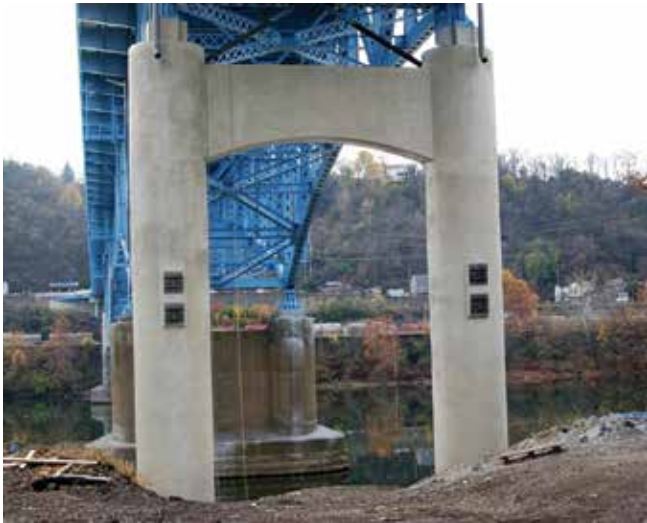
Fig. 7: Finished Rankin Bridge pier repair Photo by Dennis Bittner
