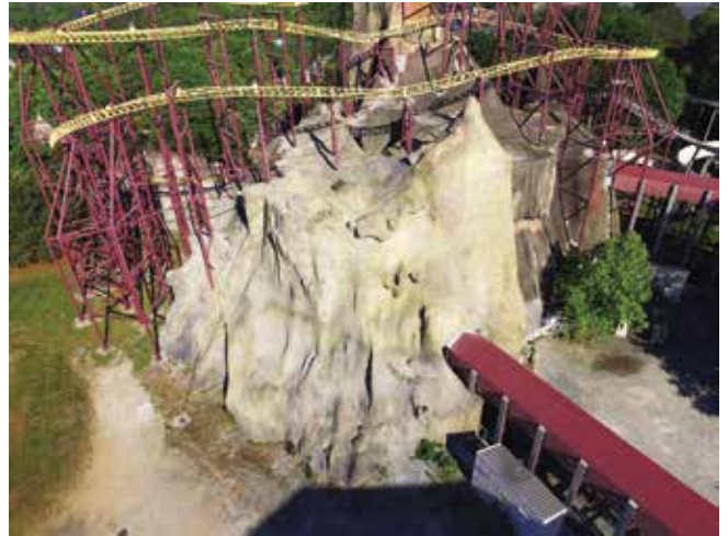
Fig. 11: Aerial view of the finished stained Kings Dominion amusement park mountain in Zone 2 and Zone 3 2016-2017 season photo by Chris Alburger
