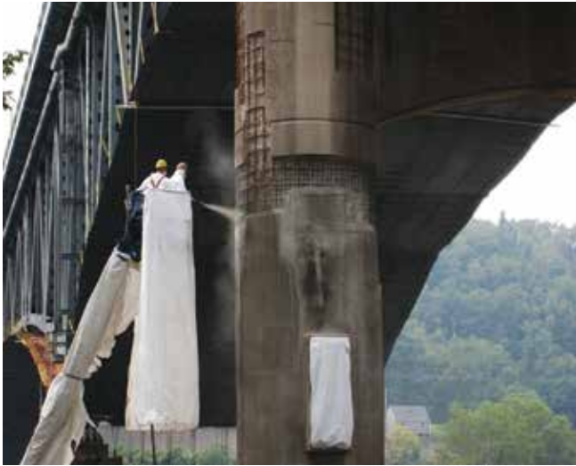
Fig. 6: Rankin Bridge pier repairs Photo by Dennis Bittner
