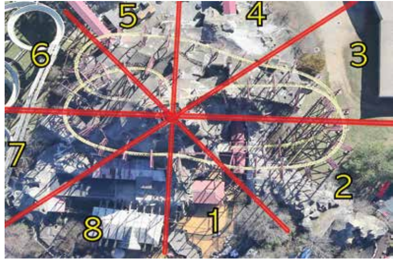
Fig. 8: The Kings Dominion amusement park volcano was divided into eight work zones for budgeting Photo by Ray Schallom
