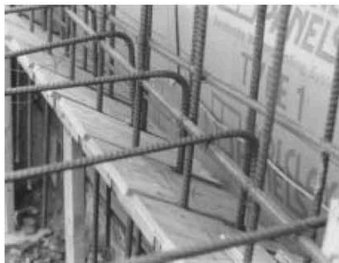
Fig. 5.1—Waterproofing panels used as back forms with wood as bottom forms.
