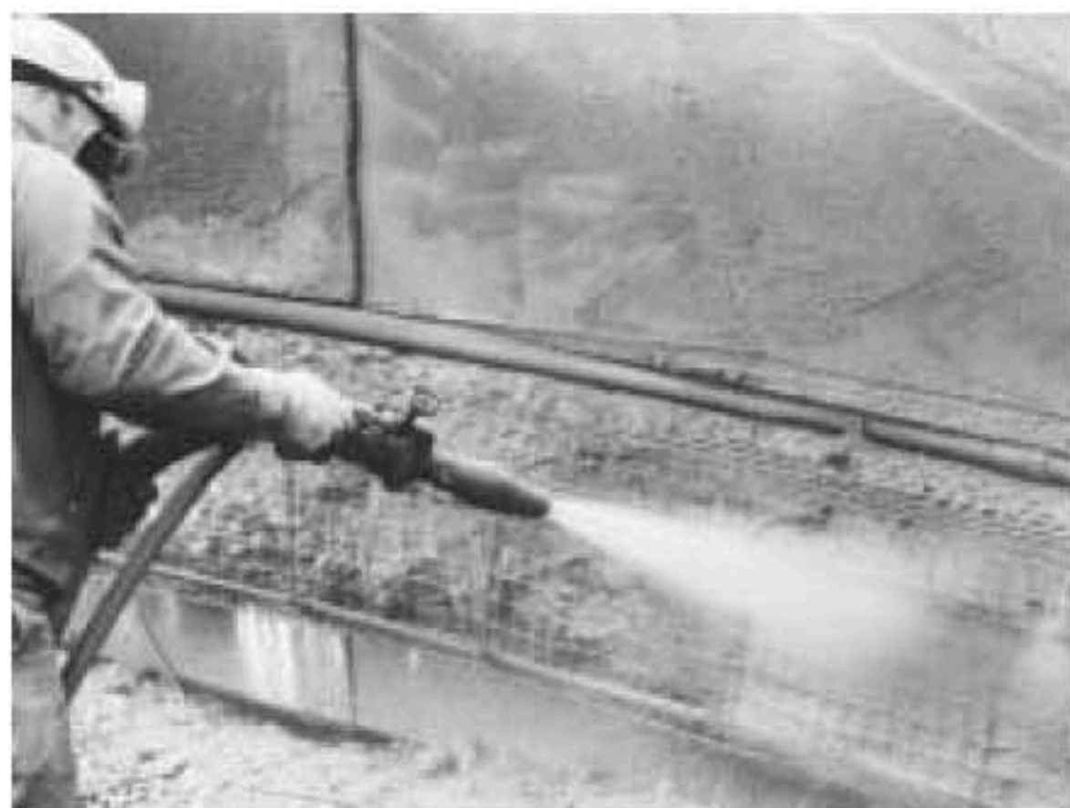
Fig. 5.2—Shooting through welded-wire mesh cut and bent to follow contours or repair.
